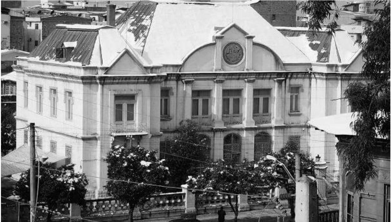
[FIGURE 14]: Former building of Babol Municipality(right). @ Taken by the researchers.
