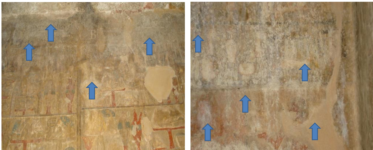
[FIGURE 9]: The deterioration of the tomb by salts and Biodeterioration effects. © Photo taken by the researcher
