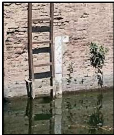
**Plate No. 35:** A Nilometer located at the eastern wall in front of the lock of the Bagouria
