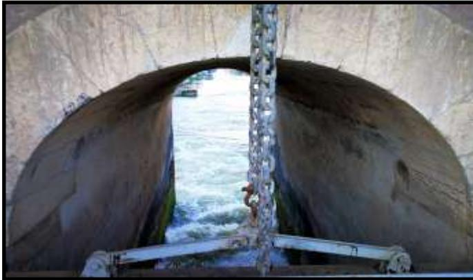
**Plate No. 4:** Tracked steel chains that carry iron gates for closing the openings of the barrage (Photographed by the researcher).
