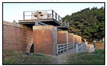
**Plate No. 8**: Viaduct and the shoulders located on the front façade of the Bagouria barrage (Photographed by the researcher).
