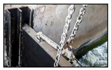
**Plate No.** 5: Recesses for the installation of iron gates of the Bagouria barrage. (Photographed by the researcher)
