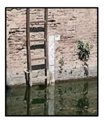
Plate No. 35: A Nilometer located at the eastern wall in front of the lock of the Bagouria (Photographed by the researcher)
